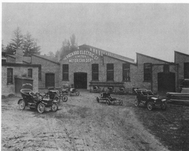
The factory buildings of the Motor Car Dept. of The Packard Electric Co., Ltd. in St. Catharines, Ontario in 1905 or 1906. In the left foreground is a completed Oldsmobile produced in this plant, while behind it are seven others in various stages of completion. The car at the right does not appear to be an Oldsmobile of any known variety. Photo from the Flummerfelt Collection, St. Catharines Historical Museum.
