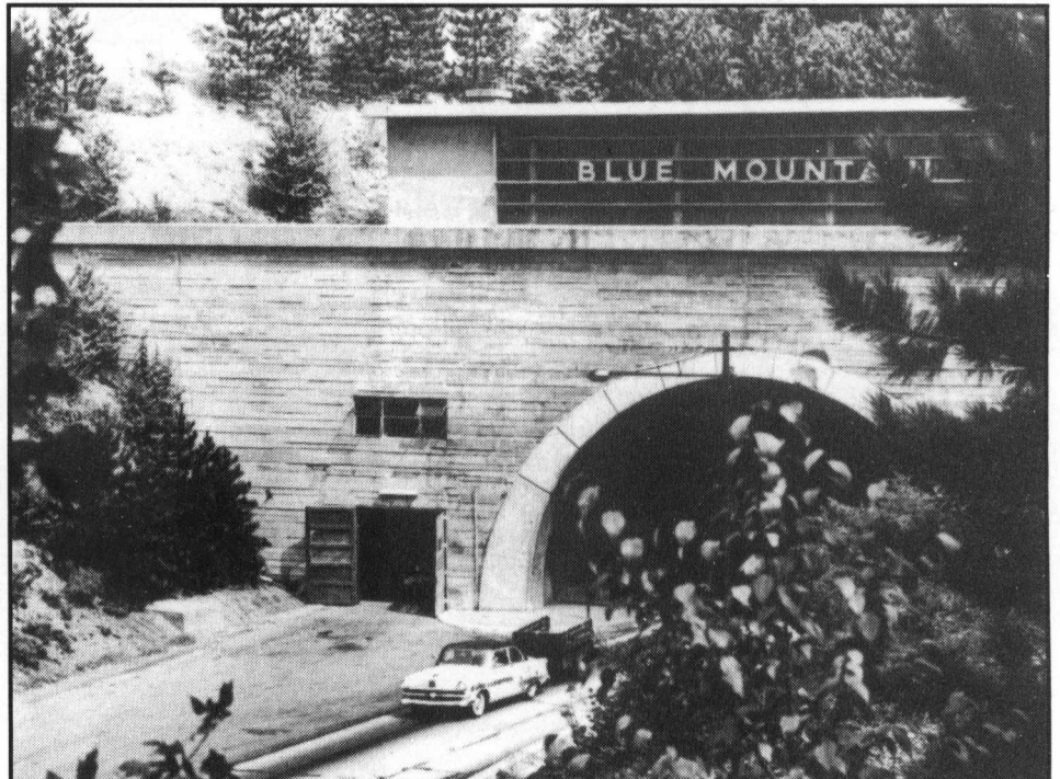
The original Turnpike utilized seven two-lane tunnels in the western Pennsylvania mountains. This is the east portal of the easternmost Blue Hill tunnel in the mid-fifties. A parallel tunnel has since increased capacity to four lanes. Pennsylvania Turnpike Commission.
