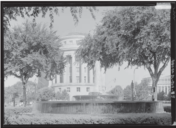
View looking to end of Federal Trade Commission Building where Constitution and Pennsylvania avenues meet; view includes the fountain built in 1950 to commemorate Andrew Mellon - Federal Trade Commission Building, Bounded by Sixth and Seventh streets, Pennsylvania and Constitution avenues, NW, Washington, District of Columbia, DC | Boucher, Jack E., creator, artist [1993]. Library of Congress.
