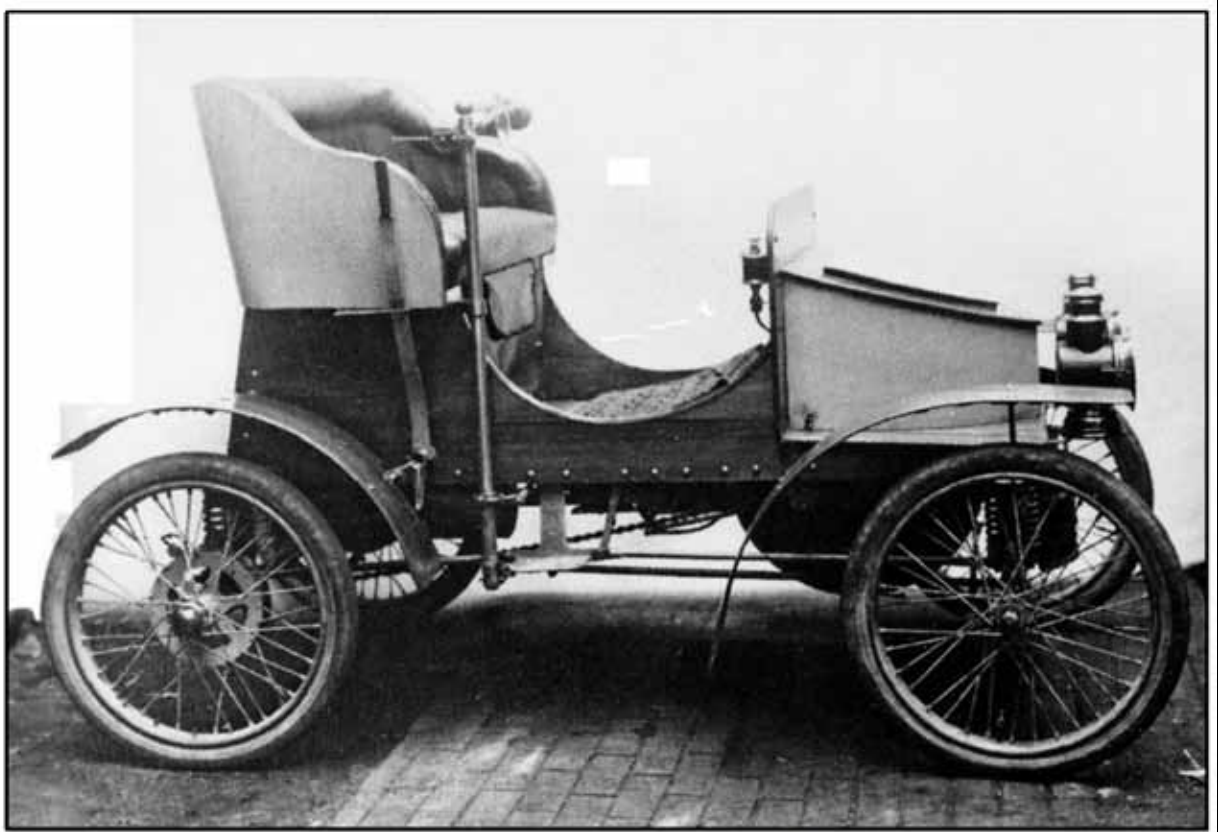
THE FIRST COMPLETED LIGHT CAR PROTOTYPE PHOTOGRAPHED AT THE VAUXHALL WORKS PRIOR TO TESTING. 09.02
