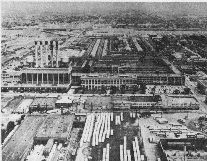
The Power Plant, left, Administration Building, center, and other buildings of Ford's Highland Park plant, birthplace of automotive mass production and the Model T, as they looked two decades ago. The powerhouse and Administration Building were razed in 1959, but the remainder of the giant factory remains in daily use.
