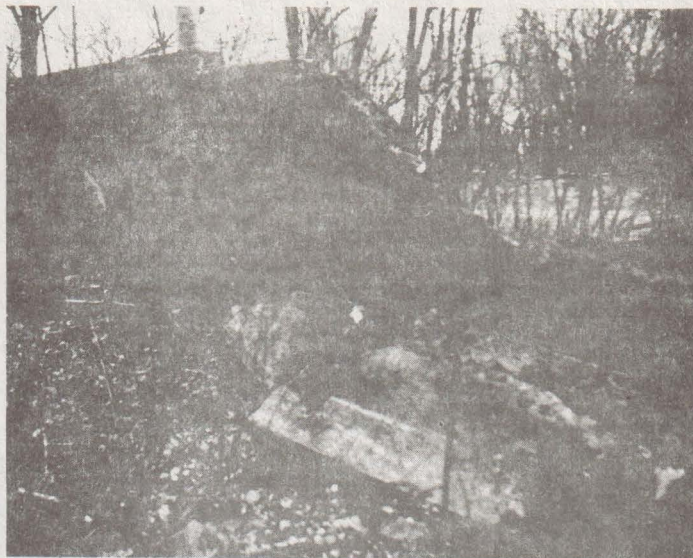
Ruins of the original Birminghams factory at Falconer, N.Y.
