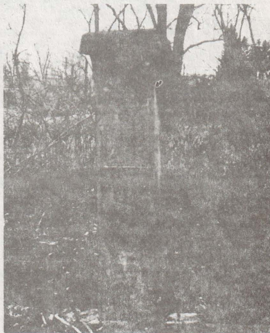
Pillar of foundation remains of the second site of the uncompleted Birminghams factory, under construction when the company went bankrupt. Located close to the R.R. tracks near factory ruins in Falconer, N.Y. The foundation was nearly 250' x 500'.
