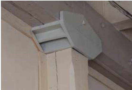
The capitals of these columns and their beveled edges are designed to frustrate the progress of flames in the event of a fire.
