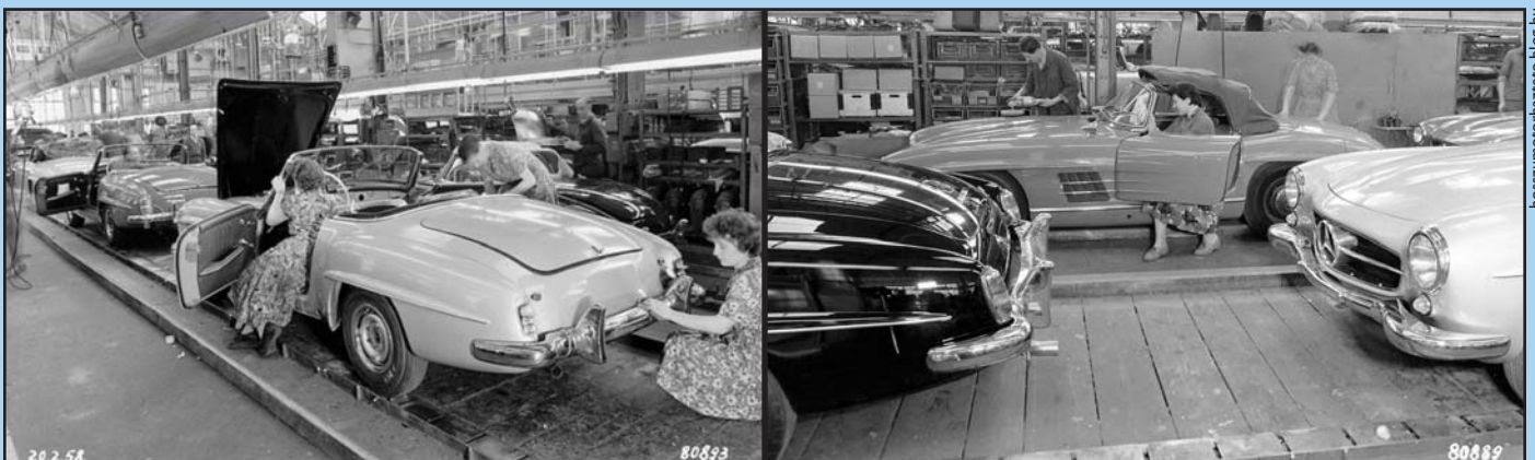
How they were made: the 190SL (model W121) in production alongside the 300SL on February 20, 1958; note the ladies in dress uniform.
