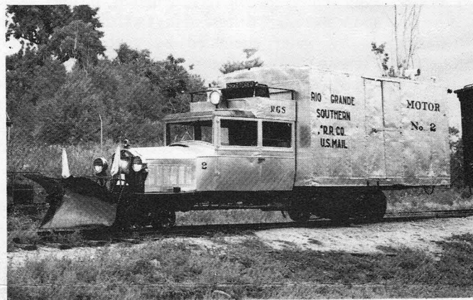
Using a 1927 Model 36 Pierce-Arrow hood and radiator, and a Buick engine, this unusual vehicle was built in 1931 by the Rio Grande Southern Railroad Company. It had a capacity of five passengers and 3,000 pounds of mail and express. Apparently it could also serve as a snowplow when the occasion demanded. It is now owned by the Colorado Railroad Museum, of Golden, Colorado.
