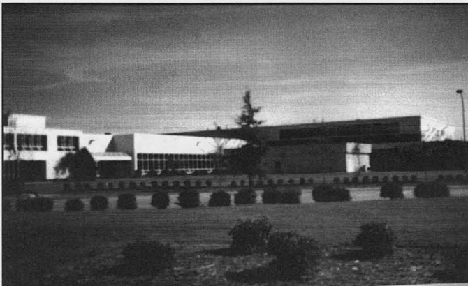
Recent photo of the former Volvo assembly plant in Chesapeake, Virginia.
