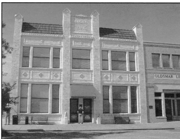
Oldsmar Bank, oldest commercial building in town (1919) is now the public library.
