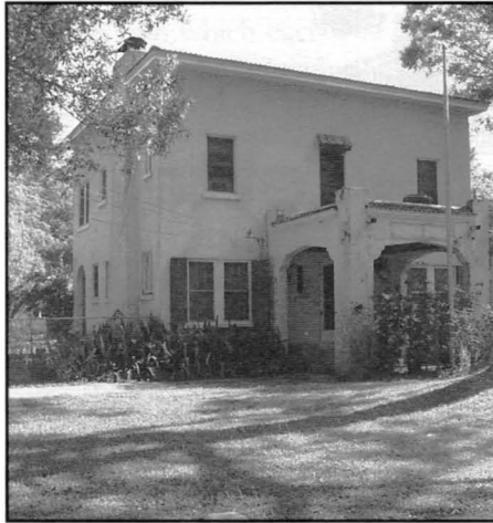
But not here. This house, designed and built for R.E. Olds, was not finished until after he had left the town.
