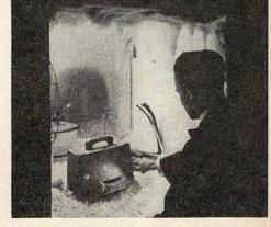
20 degrees below in test of push-button door handle. Companies have to be sure devices will work in any weather.
