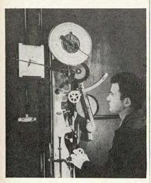
The tearing point of a piece of leather is found in this test. The pounds of pressure required to rip the piece of leather gripped between the two pincers is recorded on the chart at the left.
